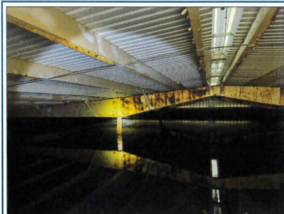
Roof Support Beams
