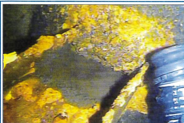
Roof Support Column at Tank Floor
