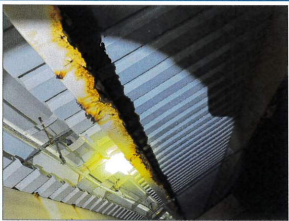
Roof Support System
