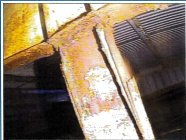
Roof Support Column at Roof Beam
