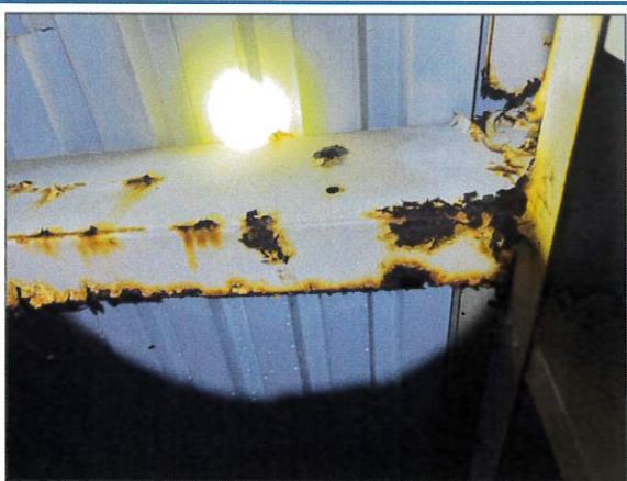
Roof Support System
